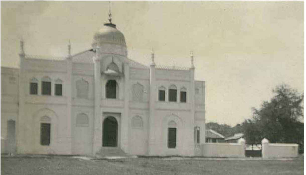
Gurdwara Sahib Silat Road after construction was just completed in 1924
