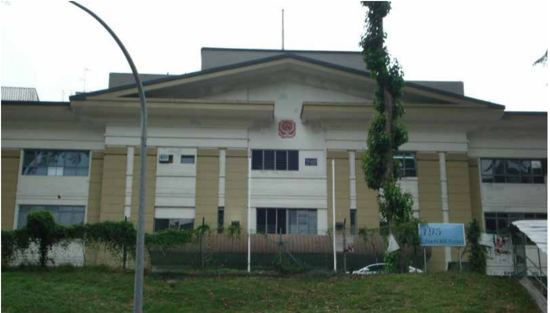
Present building on the site of the Pearl's Hill Barracks. Note the crest of the Straits Settlements Police
