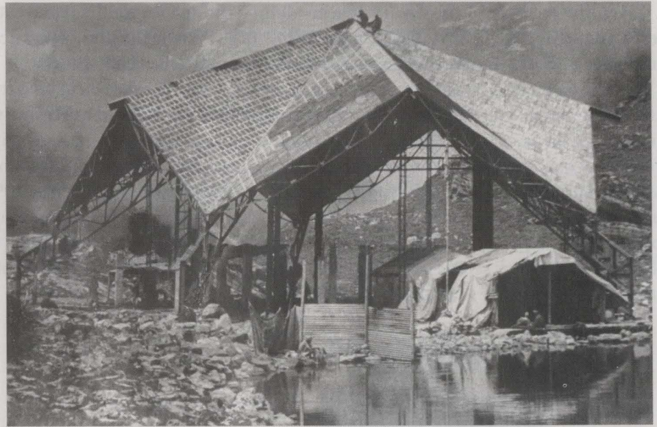
Boarding of Astrolite being laid over Steel Trusses in 1974
